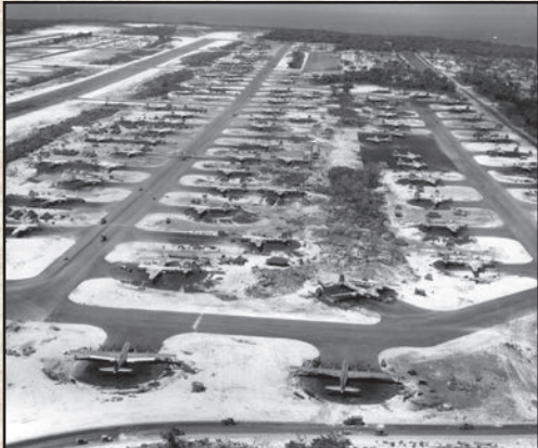
Northwest Field August 1945, View to the Northeast
